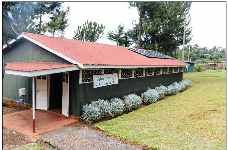
Solar Power installed in Ndubusat Health Facility
