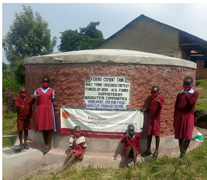
School rain water harvesting 32,000 litre tank (September 2021)
